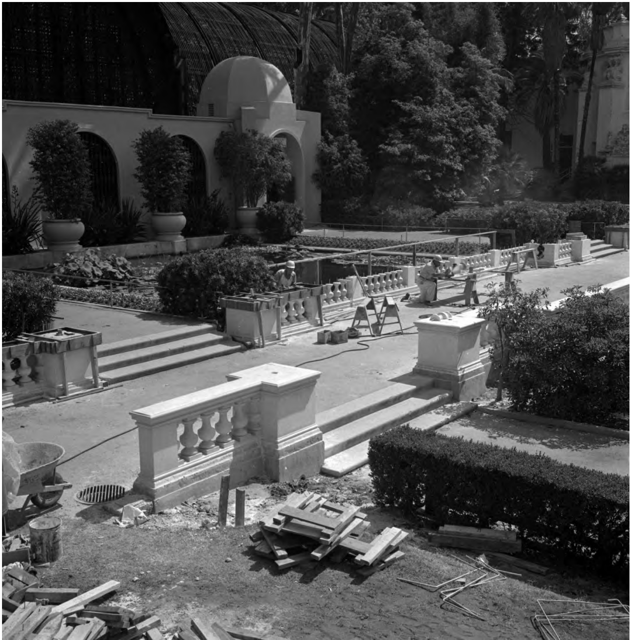
Figure 13. Reconstruction of the balustrades, facing northeast. July 22, 1964. Courtesy of the San Diego History Center, Union Tribune Collection, UT85:5212-6.
